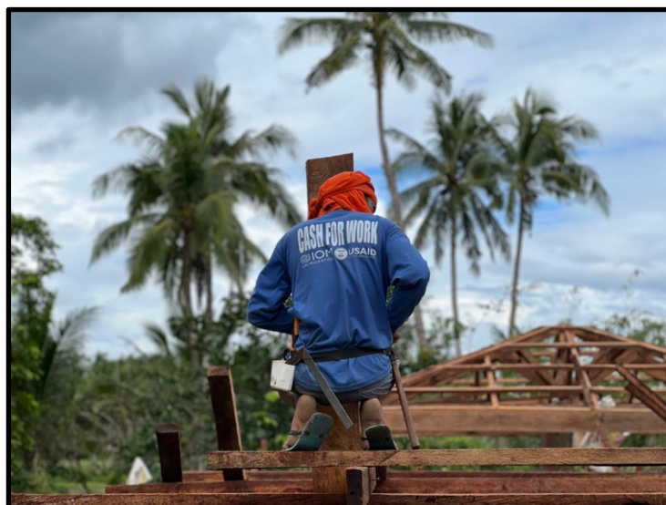
Figure 2 - Construction of evacuation center facilities (IOM, Typhoon Odette Response, 2022)
