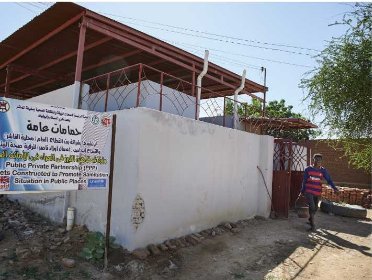
Public–private partnership toilet facility constructed to promote sanitation in the city of El-Fasher, the capital of the state of North Darfur, Sudan.
